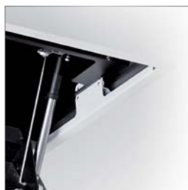
Standard ceiling finishing
